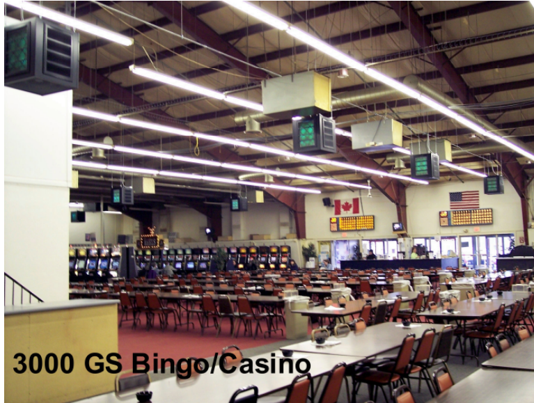
Shown without required UL shielding to block escaping UV radiation
