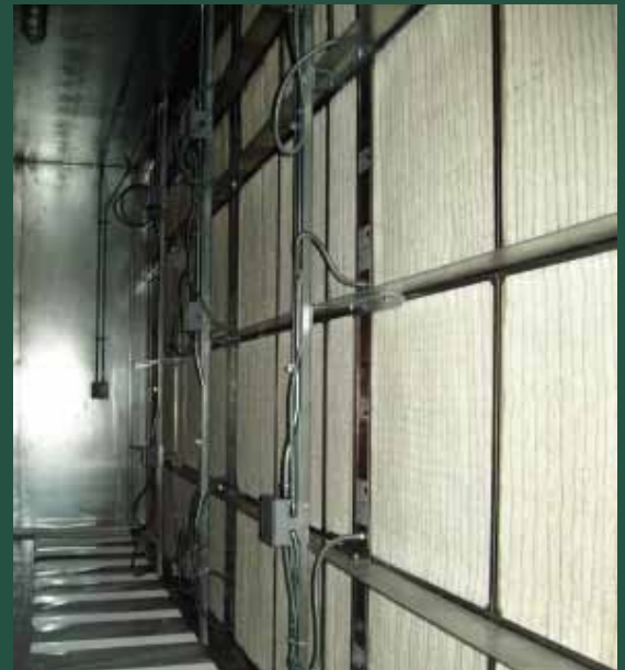
San Francisco T2 Terminal Retro-Fit
